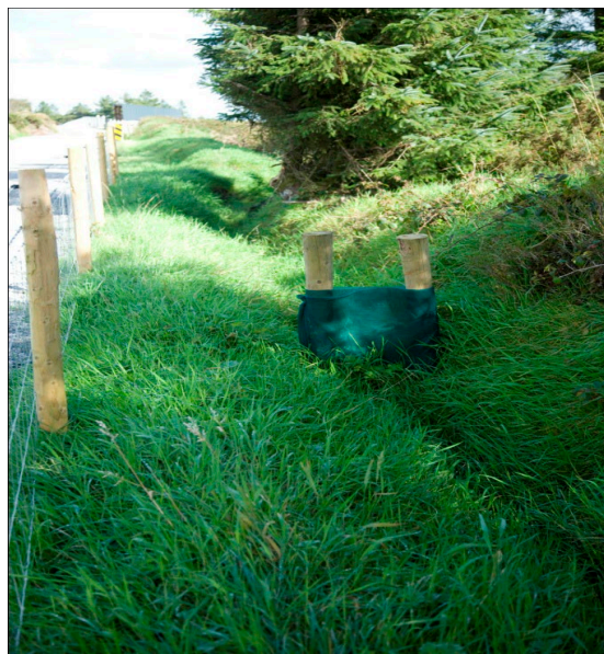
Plate 4-1: Silt trap across grassed swale
