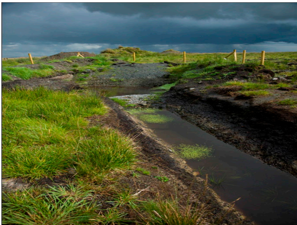
Plate 2-4: Swale draining to Settlement Pond
