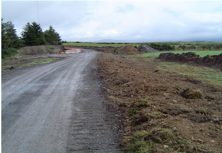
Plate 4-4: Backfill over Cable Trench
