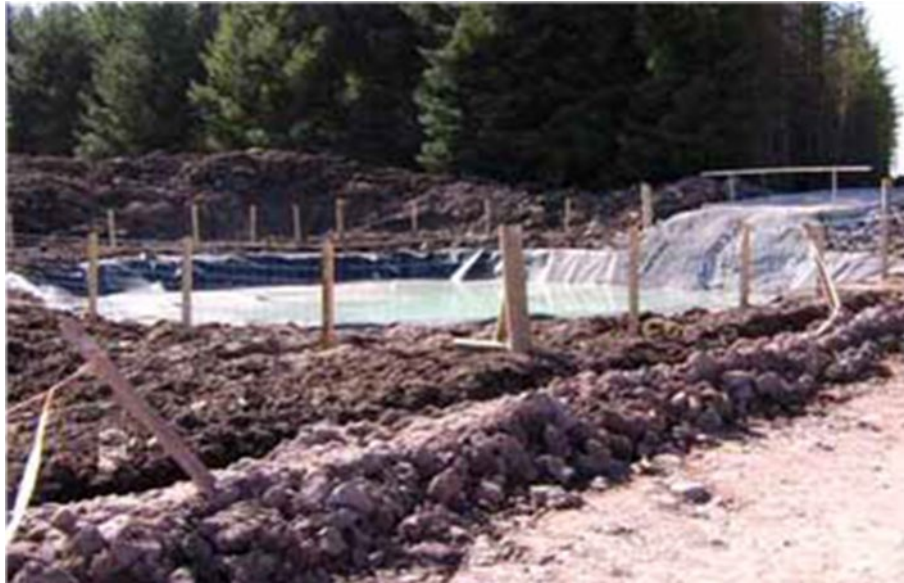
Plate 4-5: Lined Settlement Lagoon for Concrete Washout Facility
